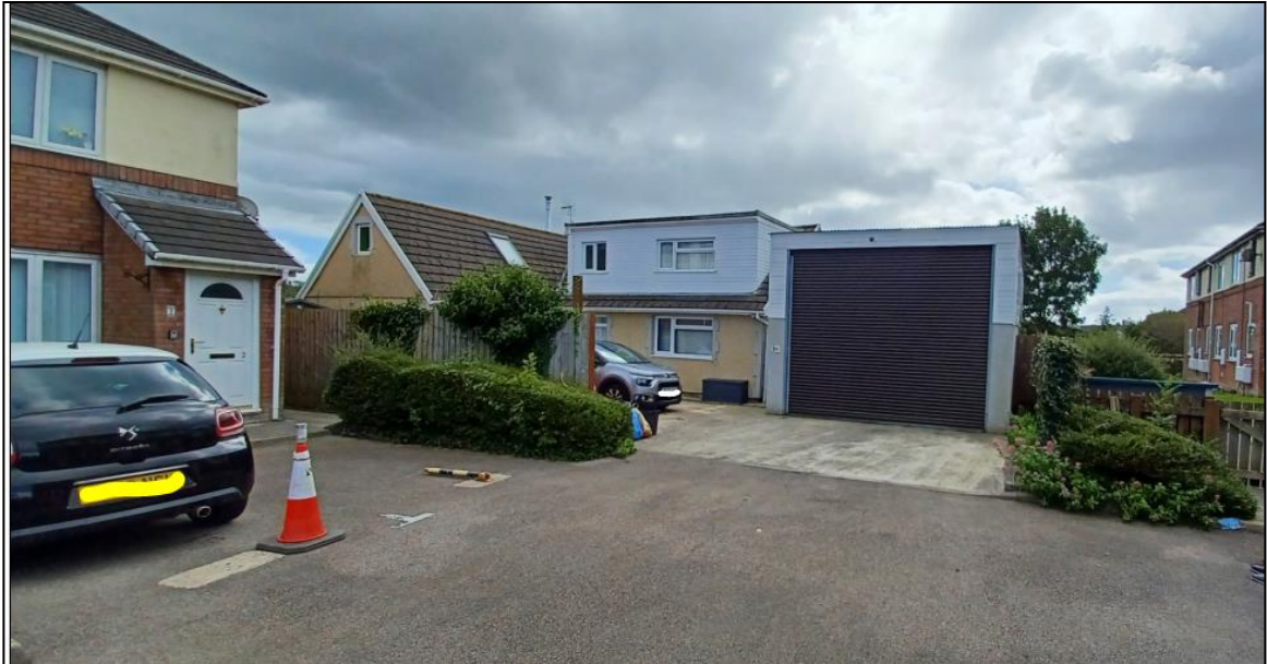
Figure 3 View of Front of Site from Greyfriars Court
