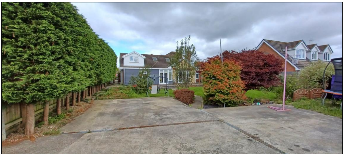
Figure 5 Rear Elevation of Application Dwelling
